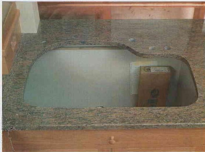
**Granite is hard but not unworkable.** Granite countertops can be made to accommodate any kitchen sink or appliance. This sink opening was roughed out with a water-cooled circular saw and then rounded and polished with hand-held grinders.
